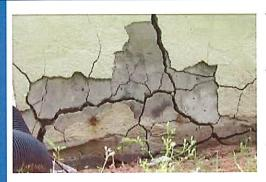
This is a reimbursement program for visual inspection and core testing for failing concrete foundations due to pyrrhotite.
