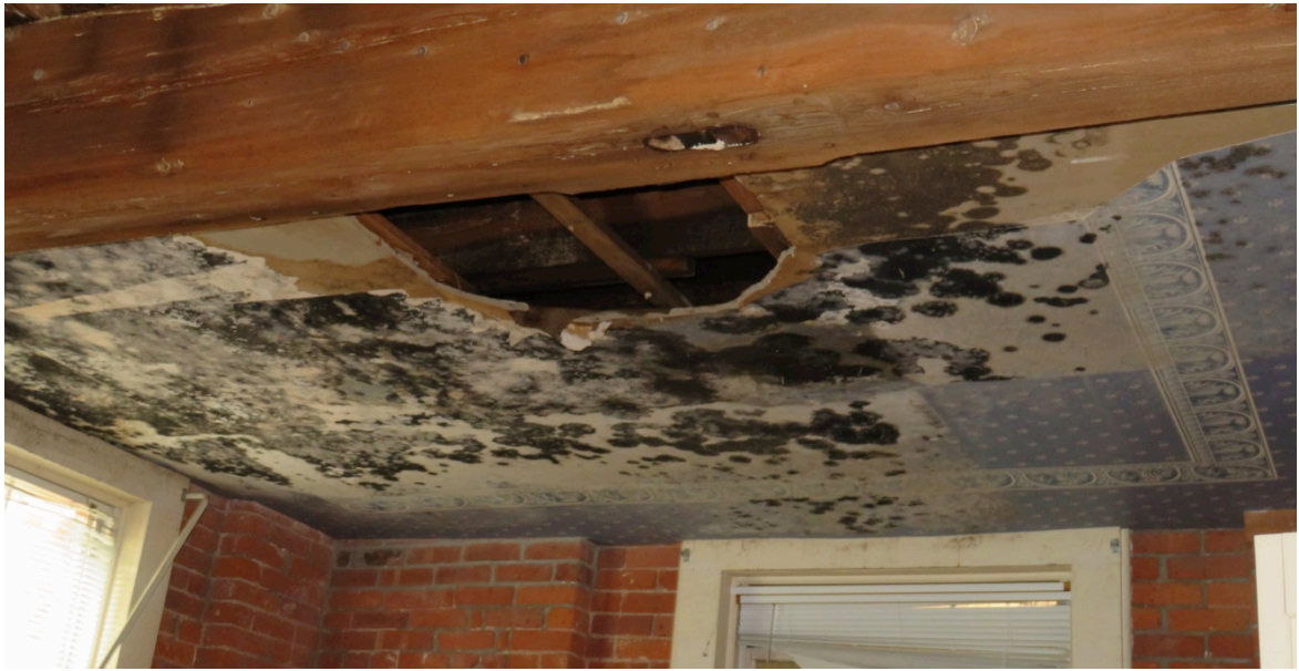
Images of Typical Mold Growth Found throughout the Building
