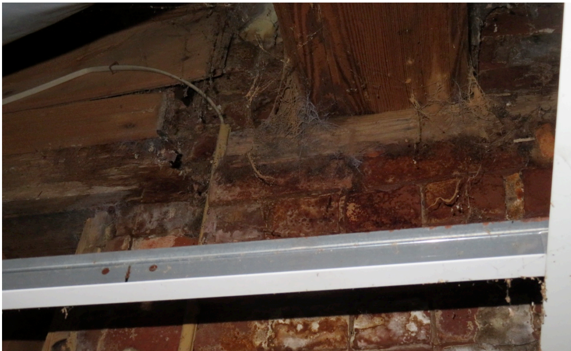
Exterior and Interior Images of Stair Tower Roof Breach Interior image shows a water-stained wood beam bearing on brick wall
