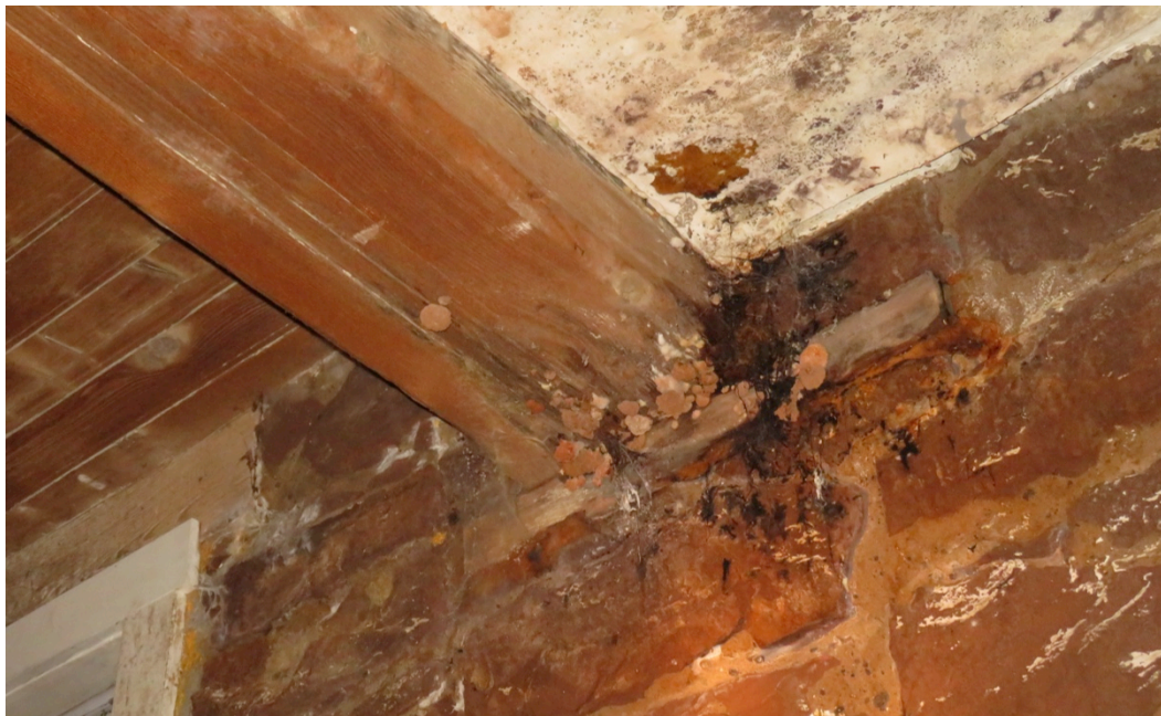
Images showing Truncated Rainwater Leader and Fungal Growth on Beam
