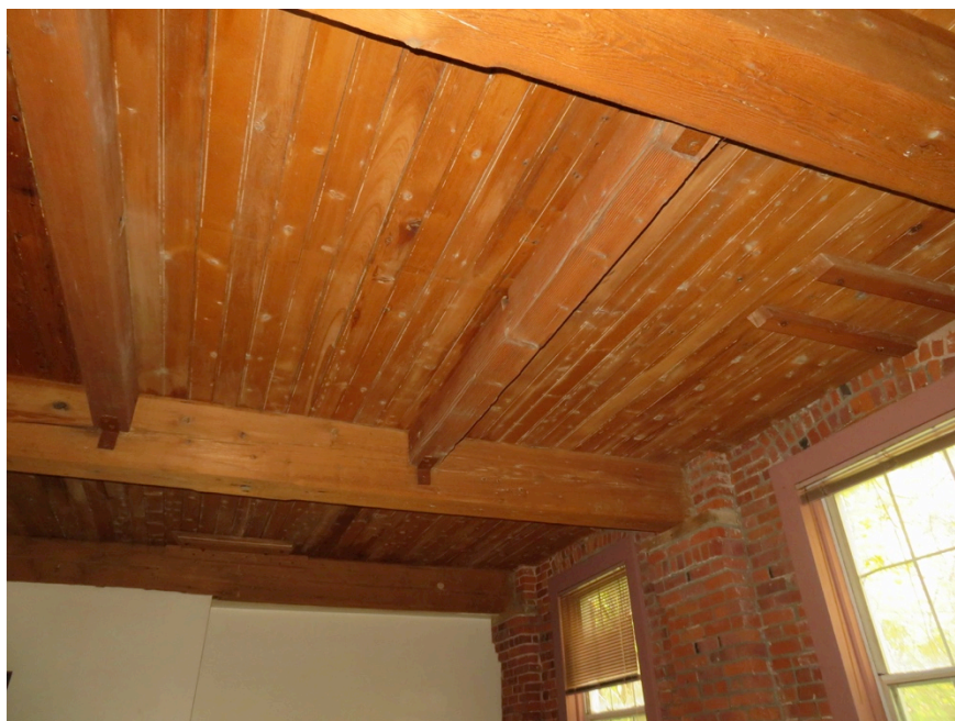
View of Typical Second Floor Framing
