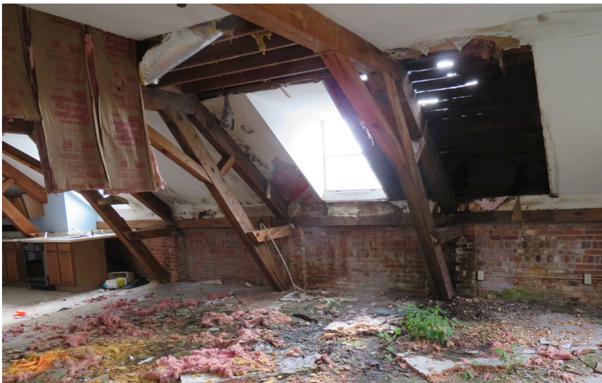
Exterior and Interior Images of West Roof Breach
