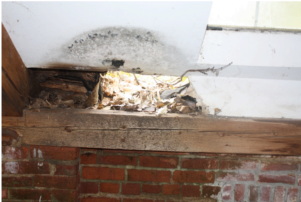
Interior Images of Opening at Cornice Breach
