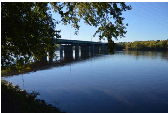
View of I-91 bridge from Town Park
