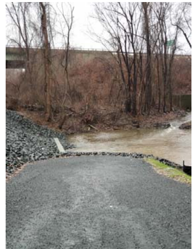
12/25/2020 Rain Event and new headwall and pipe at South Water Street
