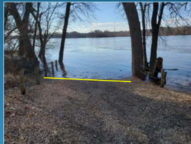
Date: December 23, 2018, noon Storm Event: 2+'' rain event Observations: Pipe under water - above flood stage river at 20-22'
