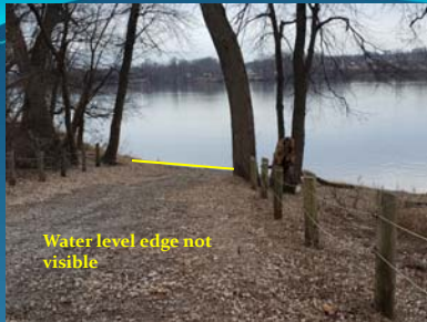
Date: December 13, 2018 Storm Event: none Timing: low flow condition - river at 10-12'+/- Location: South Water Street - Blue Ditch culverts Observations: River Flow low- discharge pipe above river elevation
