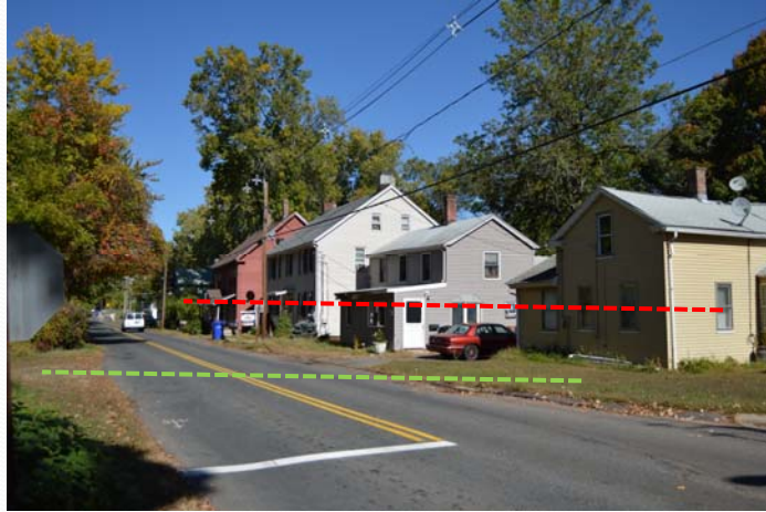
South Water Street- ROAD IS AT ELEVATION 30+/- Base Flood Elevation is 35'
