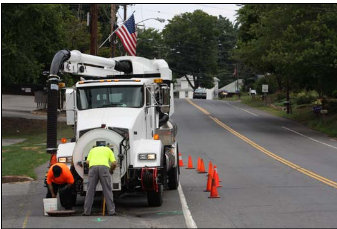
East Windsor Crew Flushing along Main Street, Broadbrook
