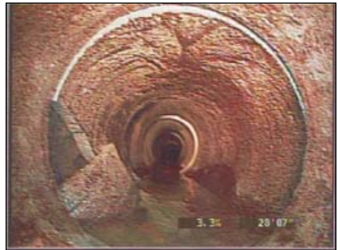
Worst case, broken pipe underground.
